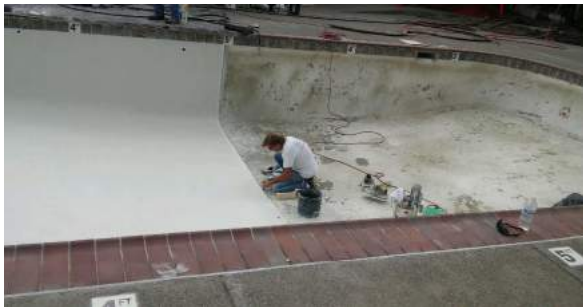
During the plastering process
