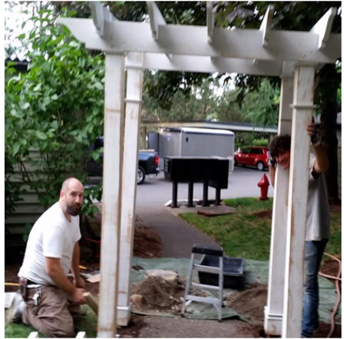
New Trellis being built! They will all be completed by August.
