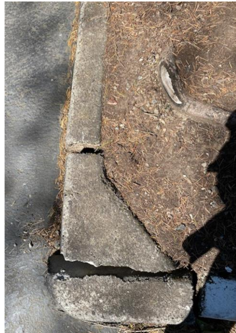
Roofing damage that is being repaired. The crane ran over the curb.
